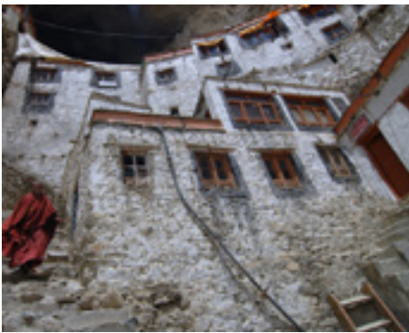
"Phuktal Monastery #1" Richard Dister, Belgium
